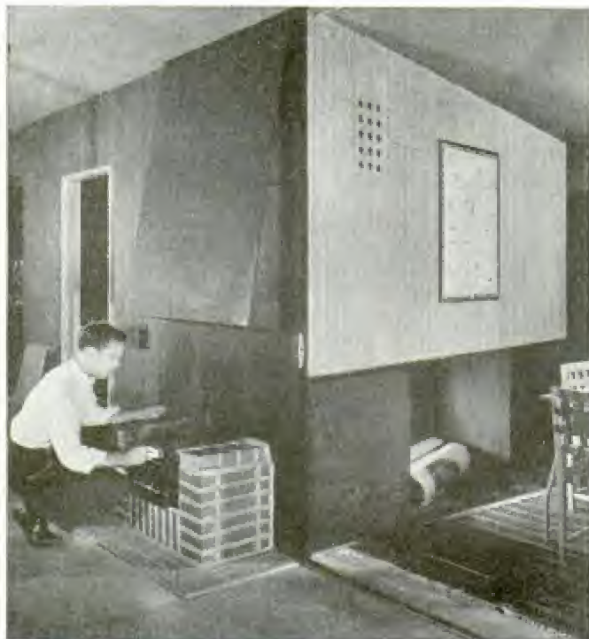
The charcoal grill and fireplace use one flue in this prefabricated "sportshack" for week ends designed by Donald Deskey
